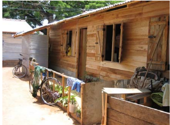
A transitional house in Kalutara, Sri Lanka, built with Australian timber. Photo: IOM Sri Lanka.
