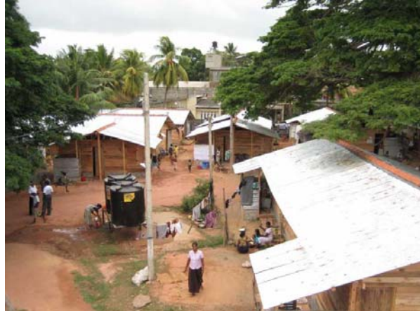
The International Organisation for Migration has used Australian timber to build this transitional housing site in Negombo, Gampaha district, in Sri Lanka. Photo: IOM Sri Lanka.
