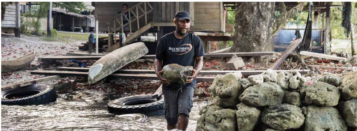
Muki Community, East Are'are, Malaita Province, Solomon Islands: Martin Hau'ato collecting rocks and building his community's sea wall that stretches across the shorelines, helping to protect homes from sea water inundation during king tides and storm surges. Credit: Ivan Utahenua, Oxfam International.
